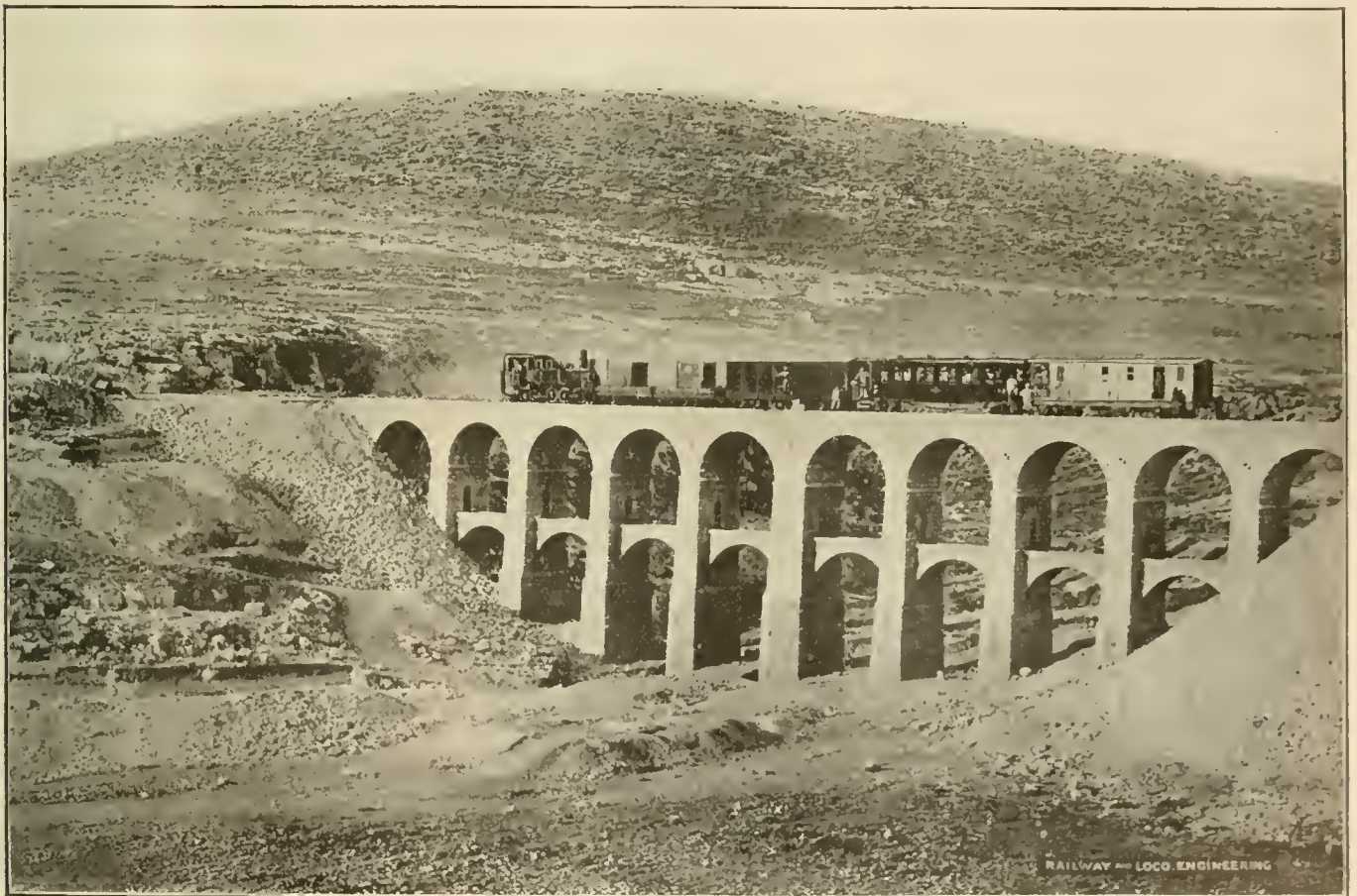
A VIADUCT ON THE DAMASCUS & MECCA R. R., NOW BEING BUILT BY TURKISH SOLDIERS, SYRIA.
